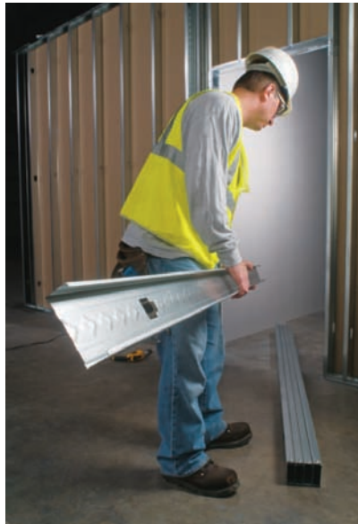
EQ-coated steel studs require the same installation methods as traditional framing products.
