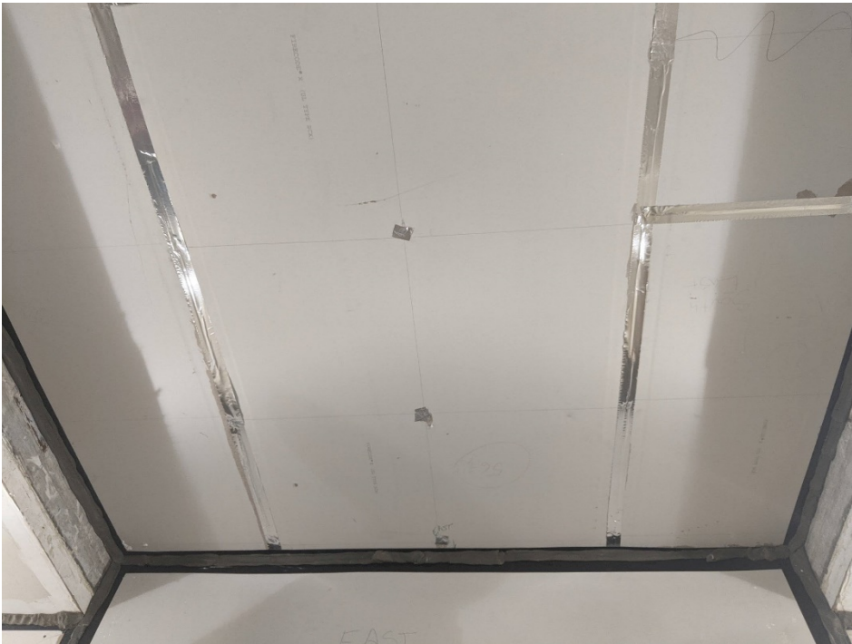
Figure 2 – Specimen mounted in test chamber, as viewed from receive room
