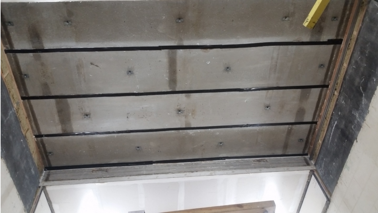
Figure 5 – Isolating clips installed to bottom of concrete slabs
