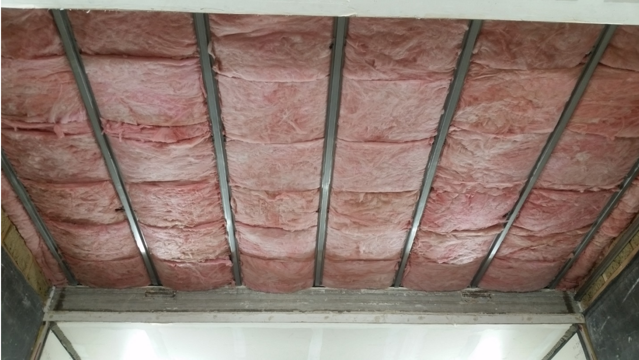
Figure 7 - Furring channel and insulation installed below slabs
