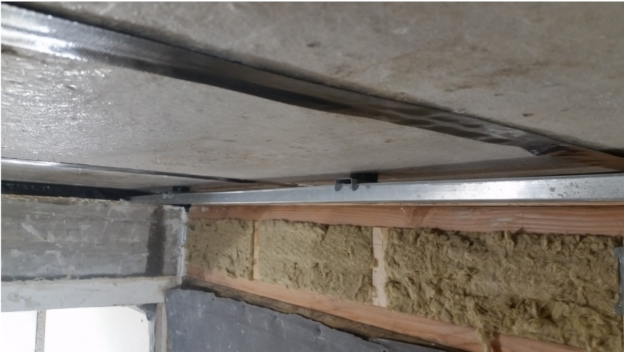
Figure 6 – Furring channel being installed to isolating clips
