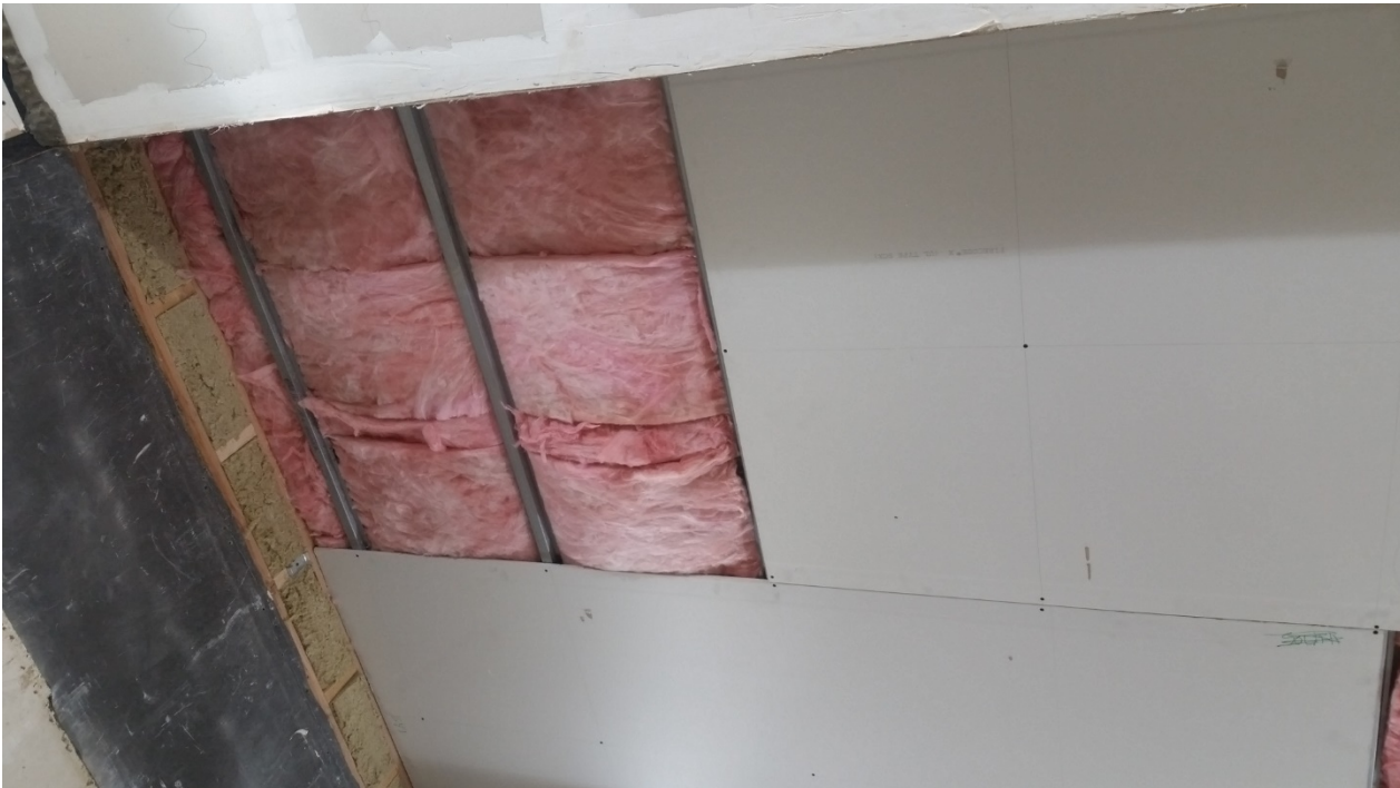
Figure 8 – Gypsum board partially installed to furring channels
