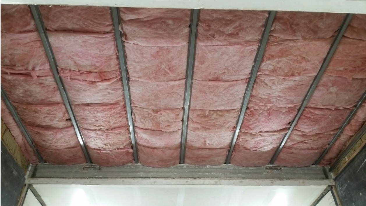
Figure 7 – Furring channels and insulation installed below slabs
