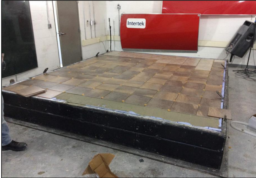
Photo No. 1 Construction of Test Specimen
