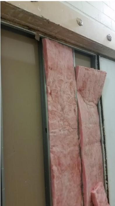
Figure 4 – Stud cavity insulation partially installed
